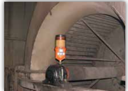
Grease lubricator installed on a blower fan
