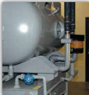
Watchdog Breather installed on a hydraulic reservoir
