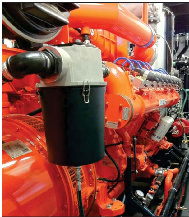
Closed Crankcase Ventilation System Guascor Engine Installation
