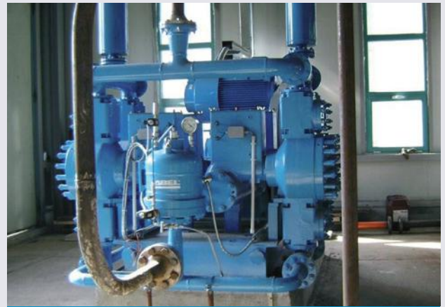
ABEL HMQ with reverse valves for transfer of fly ash with portions of coarse bottom ash
