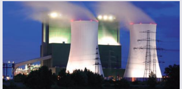
Energy/power plants – flue gas desulphurization
